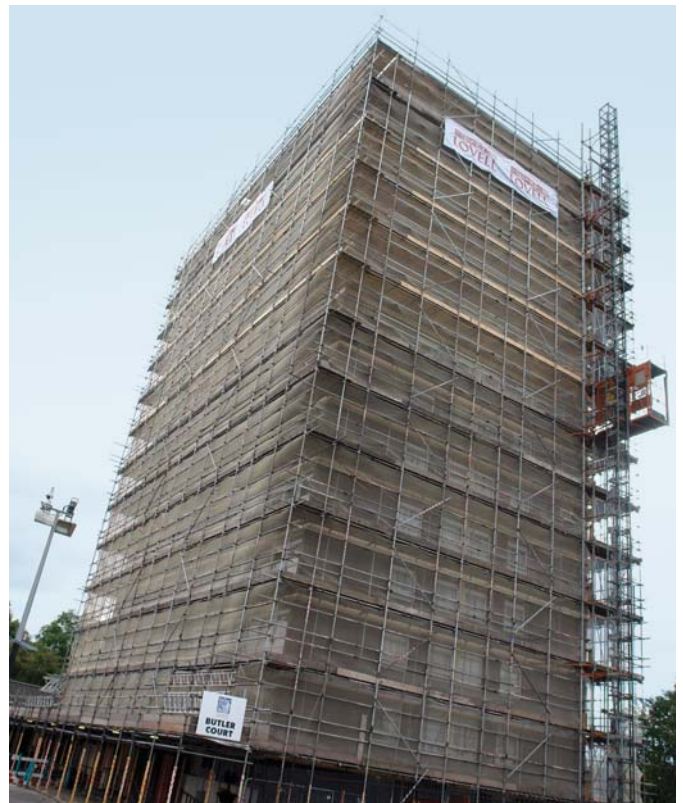
Work has started at Butler Court'
